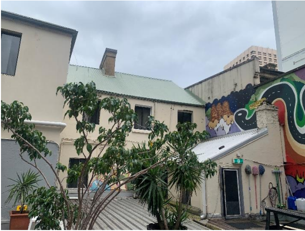
Figure 19 – View of the hostel roof terrace showing rear of 232-240 Elizabeth Street.
